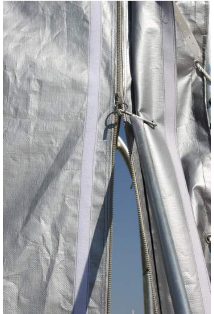
After put down door cover for front and back panel completely, using part #30 to hook the circle on the zipper in order to help opening and closing the door.
